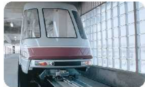
Tampa, USA INNOVIA Monorail 100 System 1991
