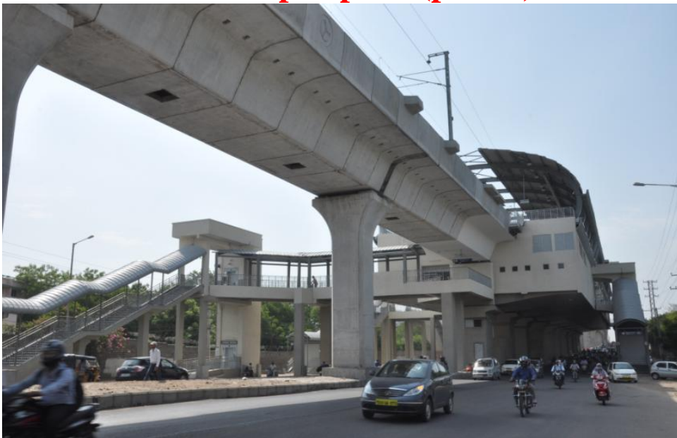
Cantilever type Metro station resting on the central pillars
