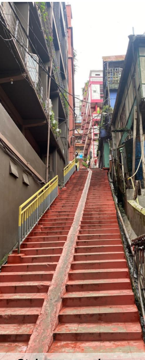
Staircases are long, steep, most are narrow and dark
