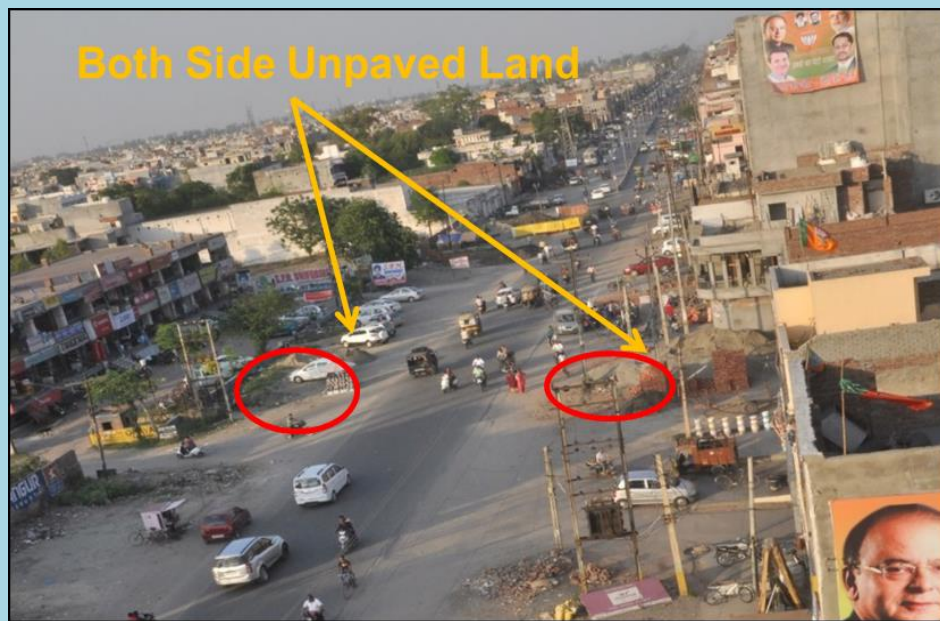
Batala Road (Before)
