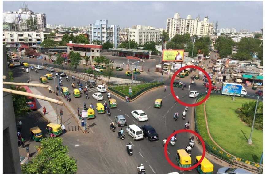
Aerial view of the junction showing conflict points
