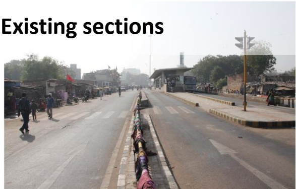
Existing condition along Patel colony to Vadaj circle
