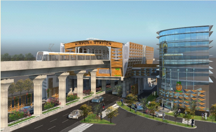
The Rs 8,680-crore project comprises two corridors with a total length of nearly 39 km. Express
