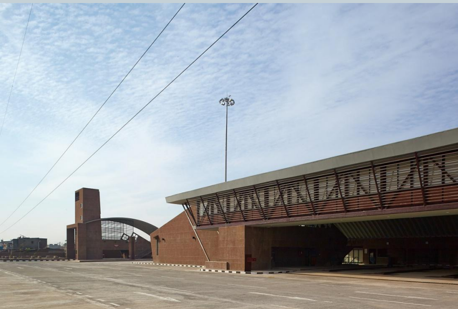
Workshop Depot, Worker's facility and bus parking
