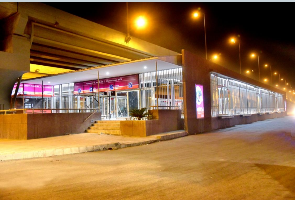
Kharwarnagar Interchange (outer view)
