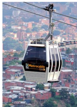
1ST INTERMODAL URBAN CABLEWAY MEDELLIN (COLOMBIA)
