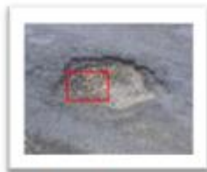
i) Detected pothole
