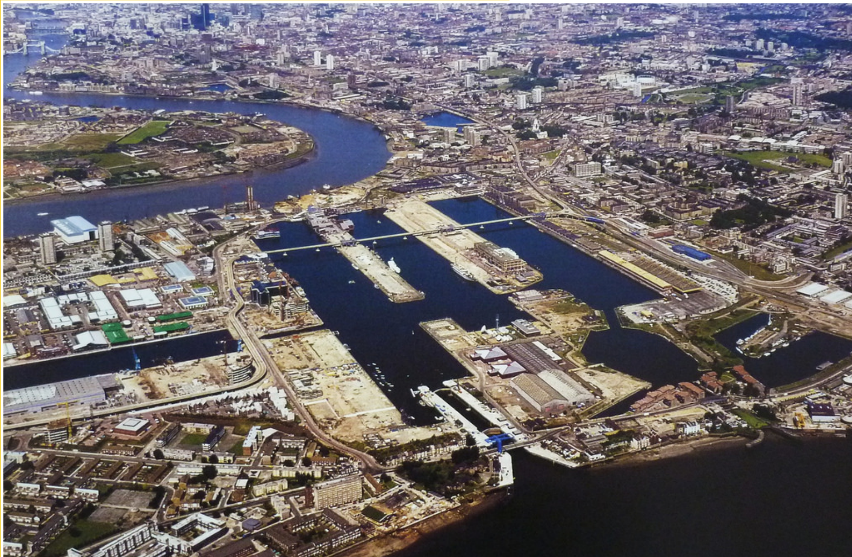
Canary Wharf Development
