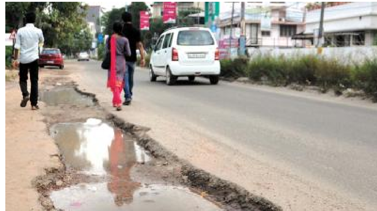
Condition of Road edges during Rainy season at Kathrikadavu
