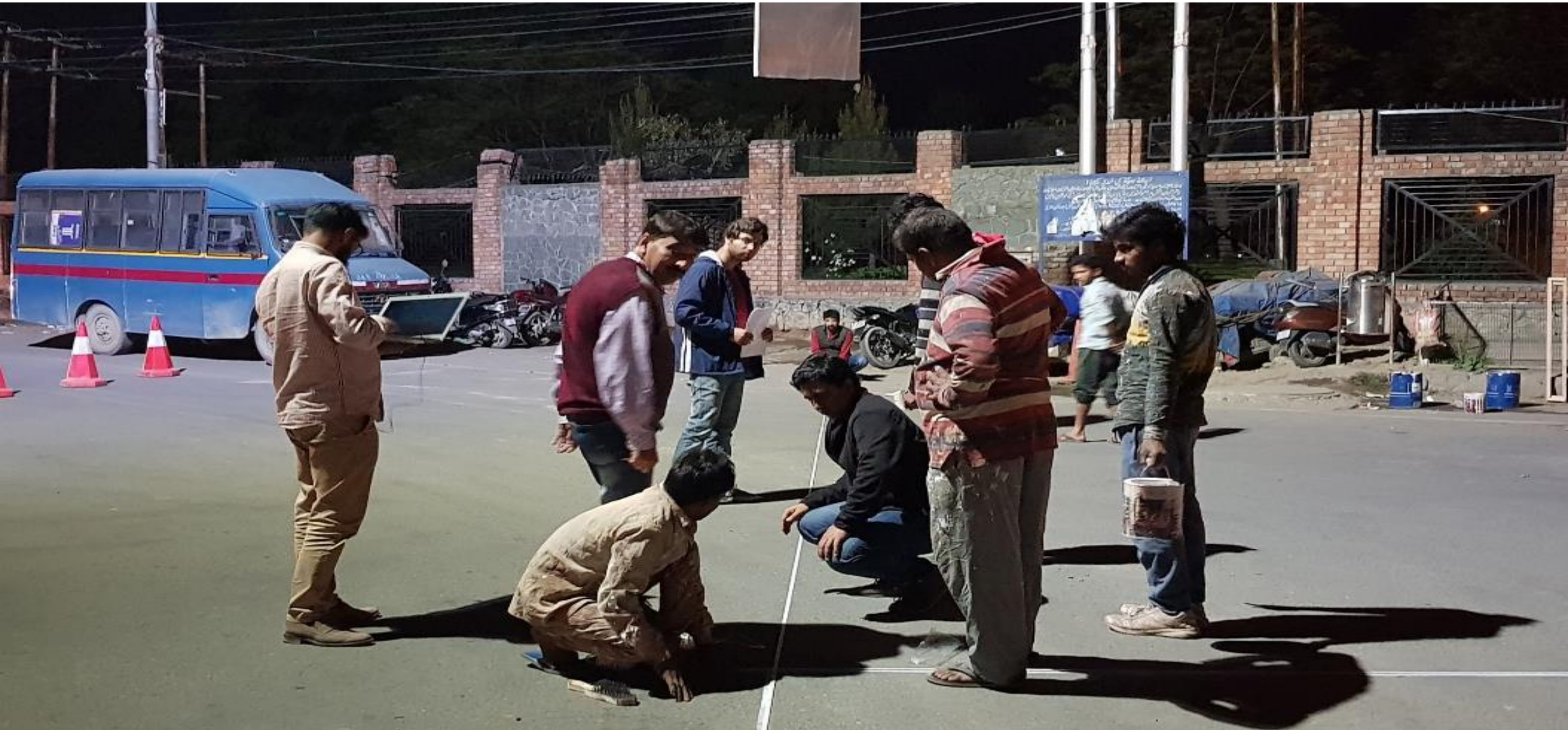
EXECUTION OF INTERVENTION DURING NIGHT
