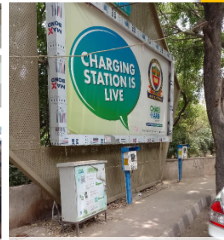
CP located on a raised curb without a ramp
