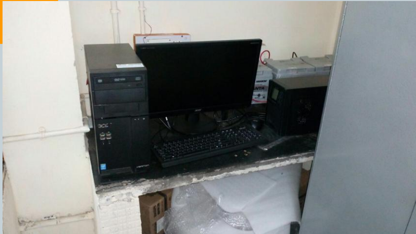
LOCATION: Bilaspur Core City Level UPTS unit at Bilaspur Municipal Corporation
