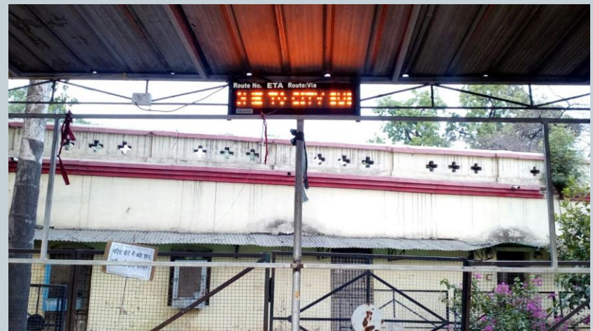
LOCATION: LED Display at Nehru Chowk, Bilaspur
