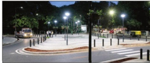
This is how St Mark's Road looks after the TenderSure work
