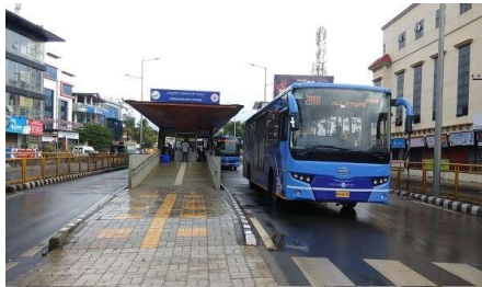
Well developed PT System
