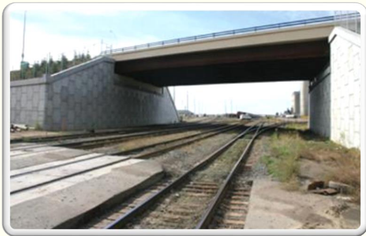
Road Over Bridges
