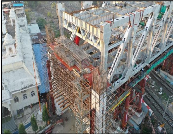
Prefab cage placing over shutters
