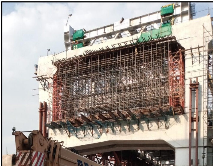
Prefab cage placing over shutters
