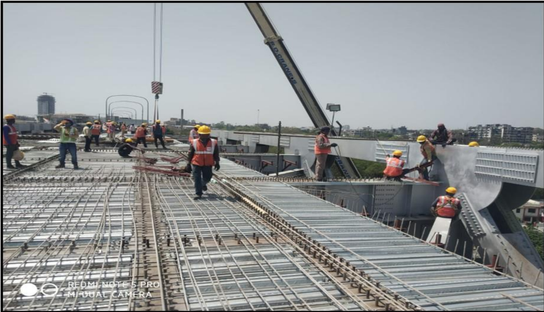
Deck Slab Construction of Steel Truss
