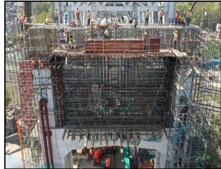
Balance reinf. Fixing and side shuttering
