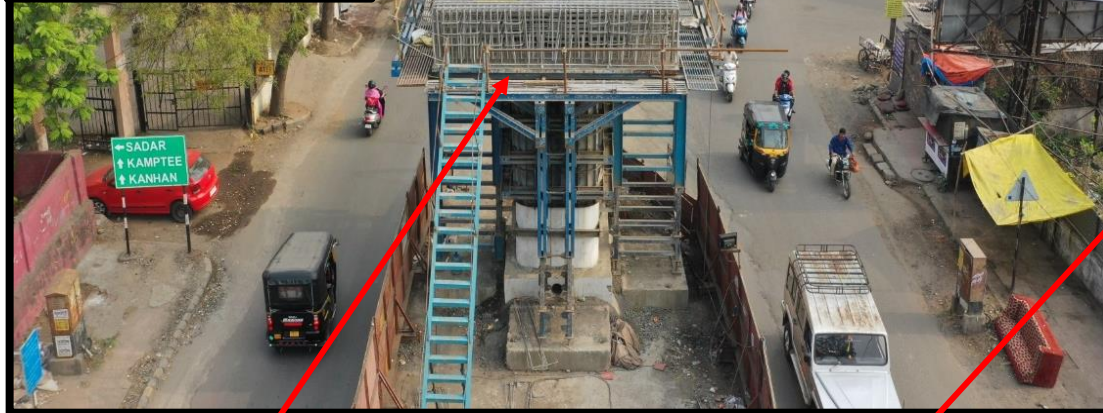
Construction of Flyover Level Pier Cap
