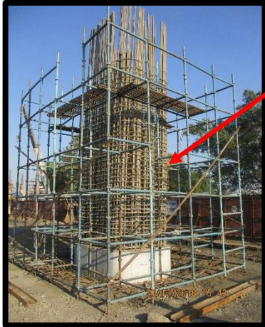
Construction of Flyover Level Pier
