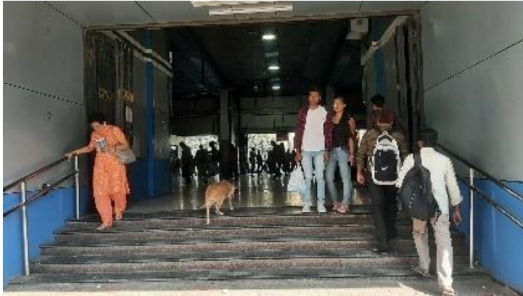
Absence of tactile provisions; handrail provisions not as per standards
