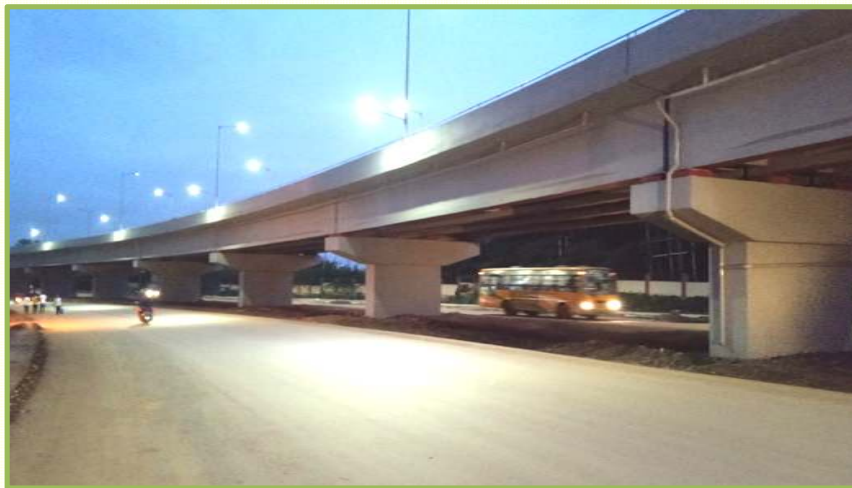
GRADE SEPERATOR NAVANAGAR
