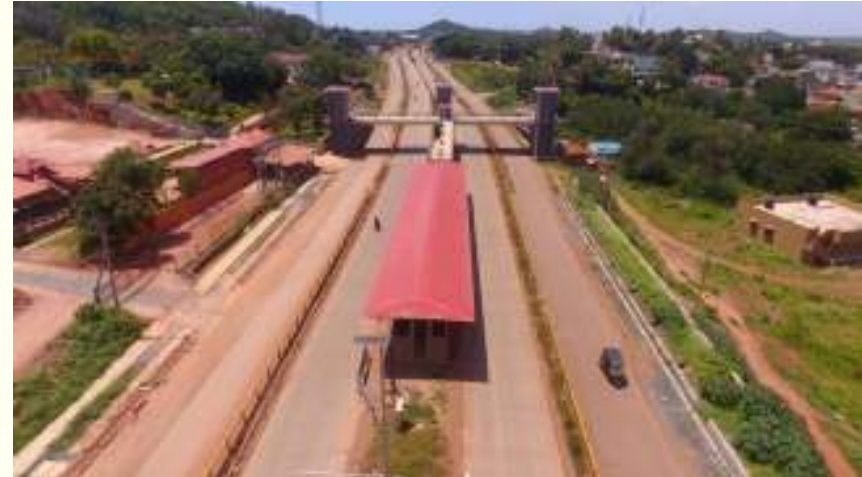
44 MTR CORRIDOR AT BUS STATION LOCATION
