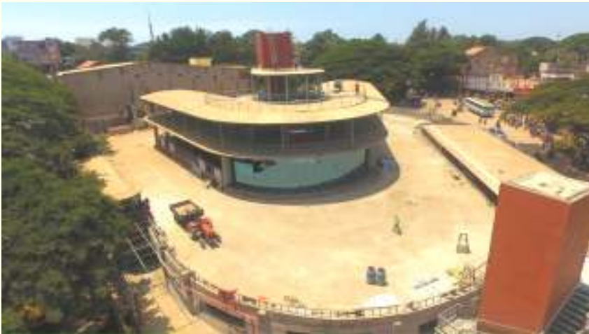
BRTS TERMINAL DHARWAD MITRASAMAJ
