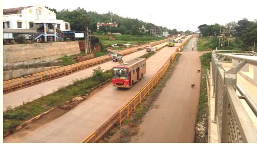
FIXED RAILINGS IN BETWEEN BRTS AND MTL CORRIDOR
