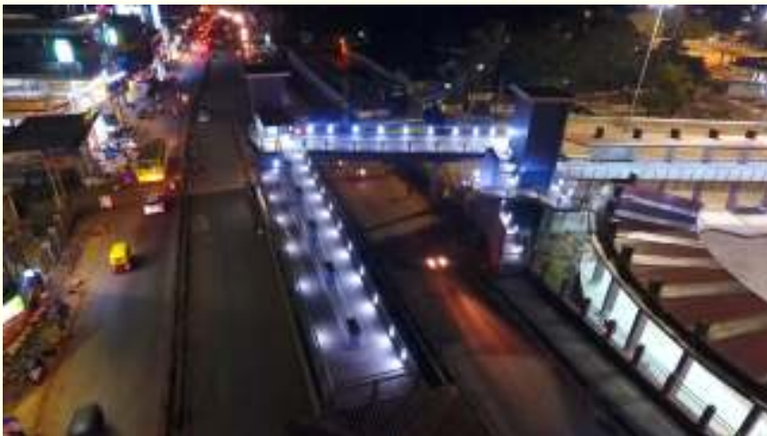
FOOTOVER BRIDGE AT NIGHT VIEW
