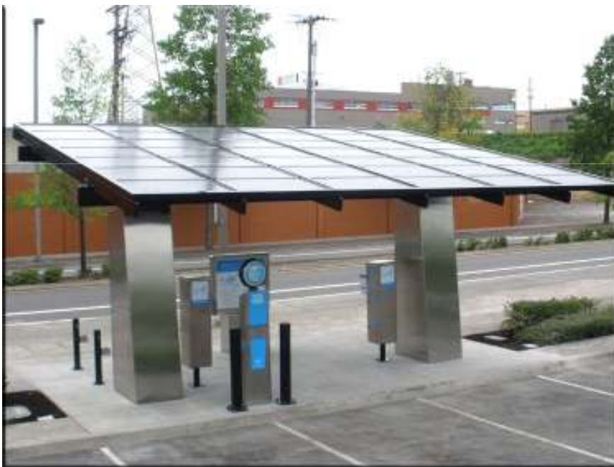
Solar-Powered Electric Vehicle Charging Station, Debut, Portland.
