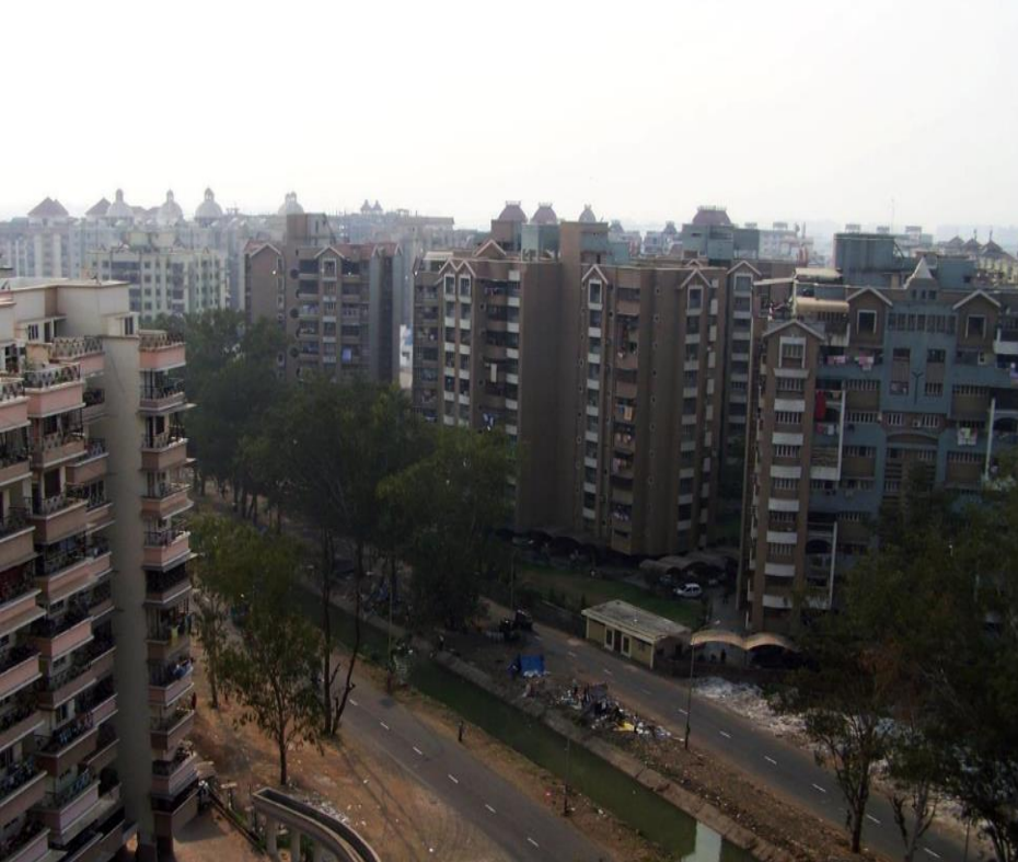
Under maintained Canal diving the City
