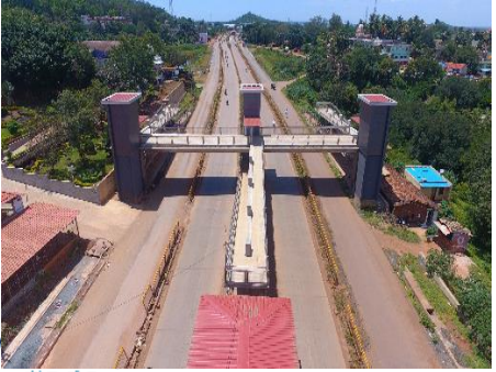
Foot Over Bridges for BRT Station
